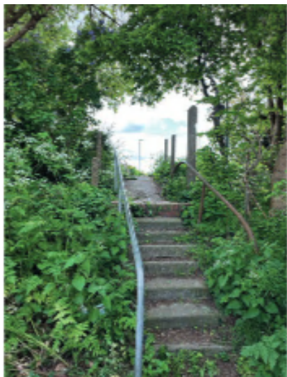
View A - Looking up the path to Rose Cres.
